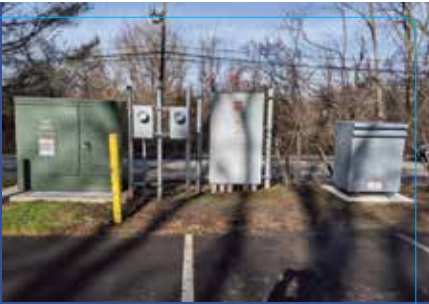
The solar energy system interconnects with PECO's distribution grid and the St. Thomas buildings . One meter measures the electricity generated and the other meter measures electric usage. Excess generation goes onto the grid and results in a credit to St. Thomas.
