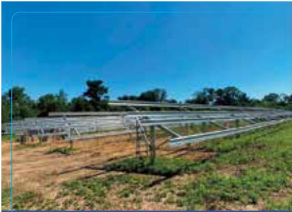
The Solar Racking System that supports the panels points due South and is fixed at a 25° angle to the ground. The land under the panels has been planted in no-mow grass to reduce grounds maintenance costs.
