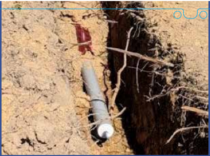
Underground Conduit houses the wiring used to carry the Alternating Current from the inverters at the solar field to the utility interconnection site in the parking lot below St. Thomas' Preschool.
