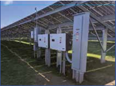
Two 125kW String Inverters convert the Direct Current (DC) output from the solar modules into Alternating Current (AC) that is used by St. Thomas' buildings and by the PECO grid.
